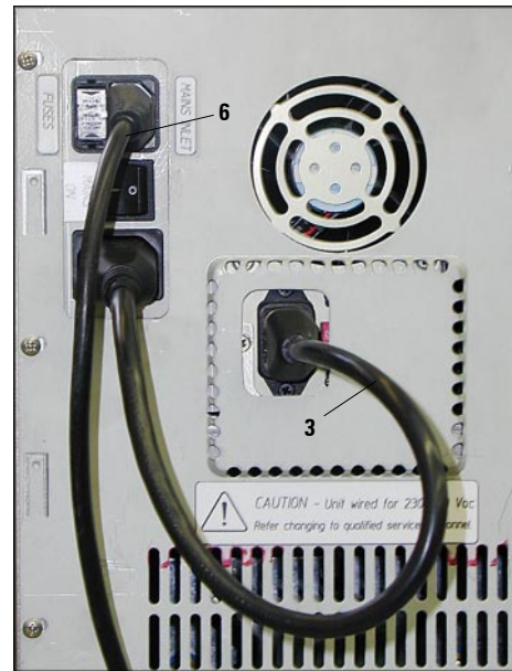
Fig. 3 Cables connected correctly
